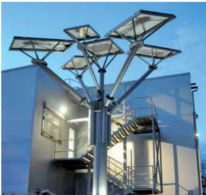
"Tree" with solar panels, installed at the Network Operations Center in Busines Park Sofia
